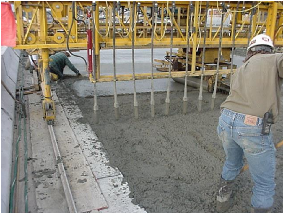
Figure 3: Vibrator used on Morgan Bridge Deck
