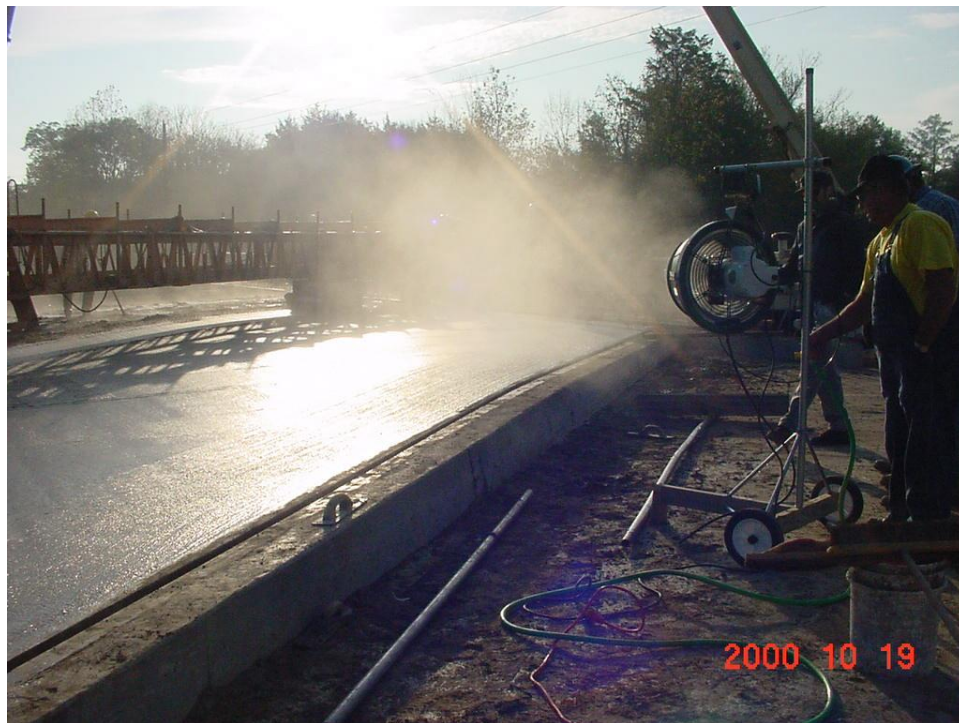
Figure 1: Fogger used on Adona Bridge Deck
