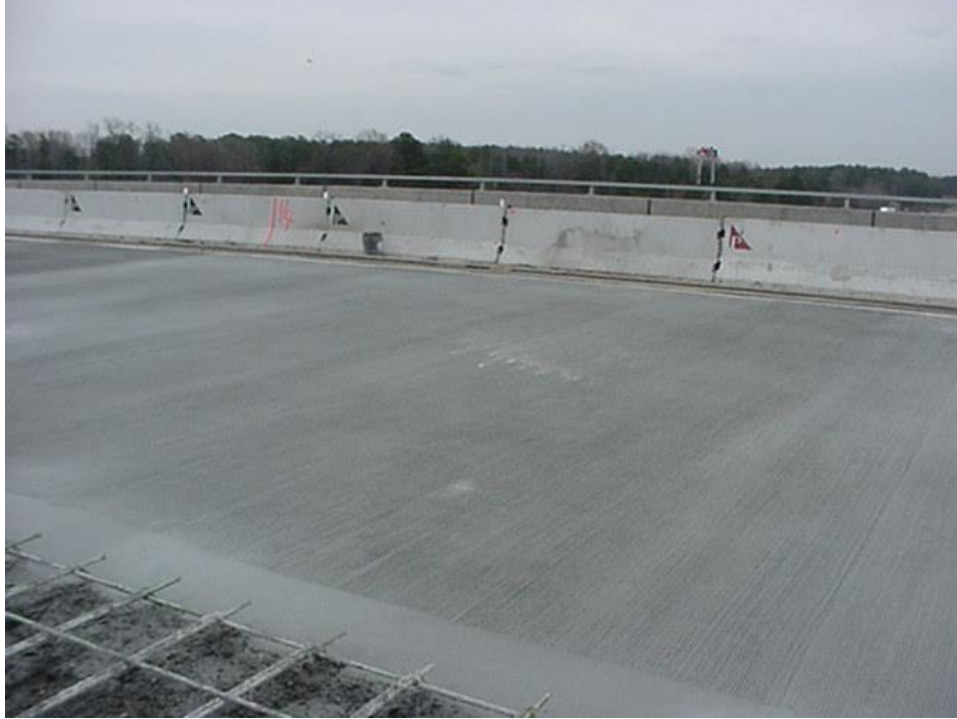
Figure 4b: Tining on Morgan Bridge Deck
