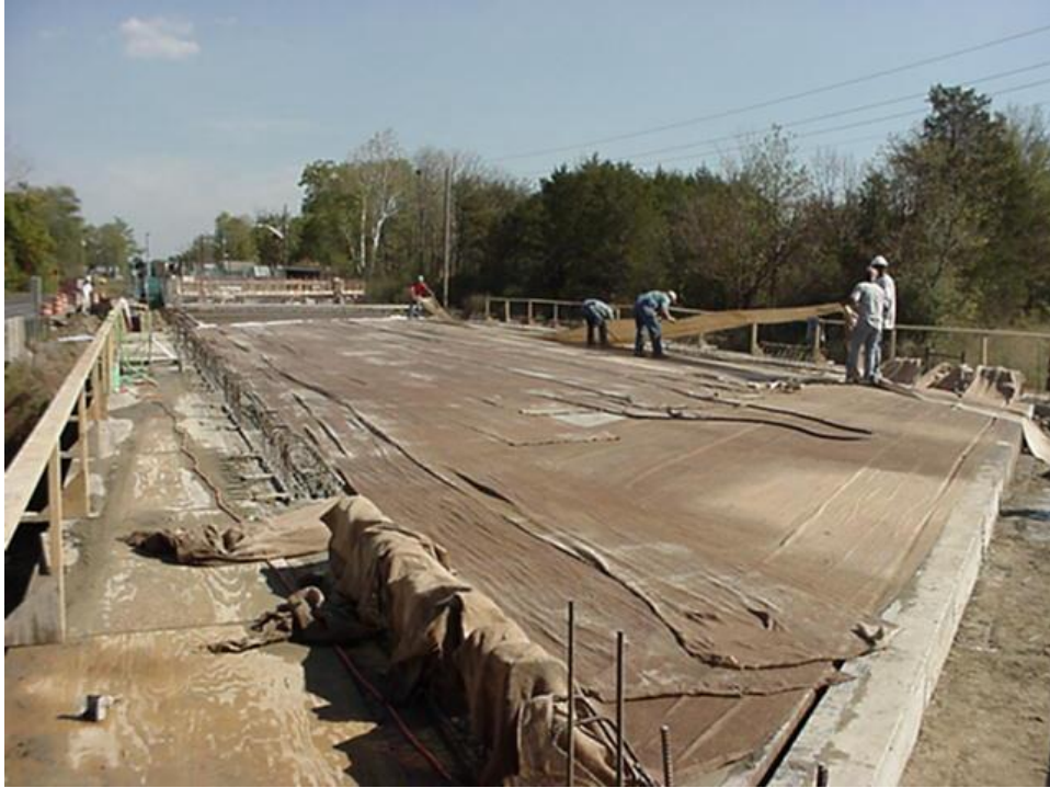
Figure 2: Burlap Curing on Adona Bridge Deck
