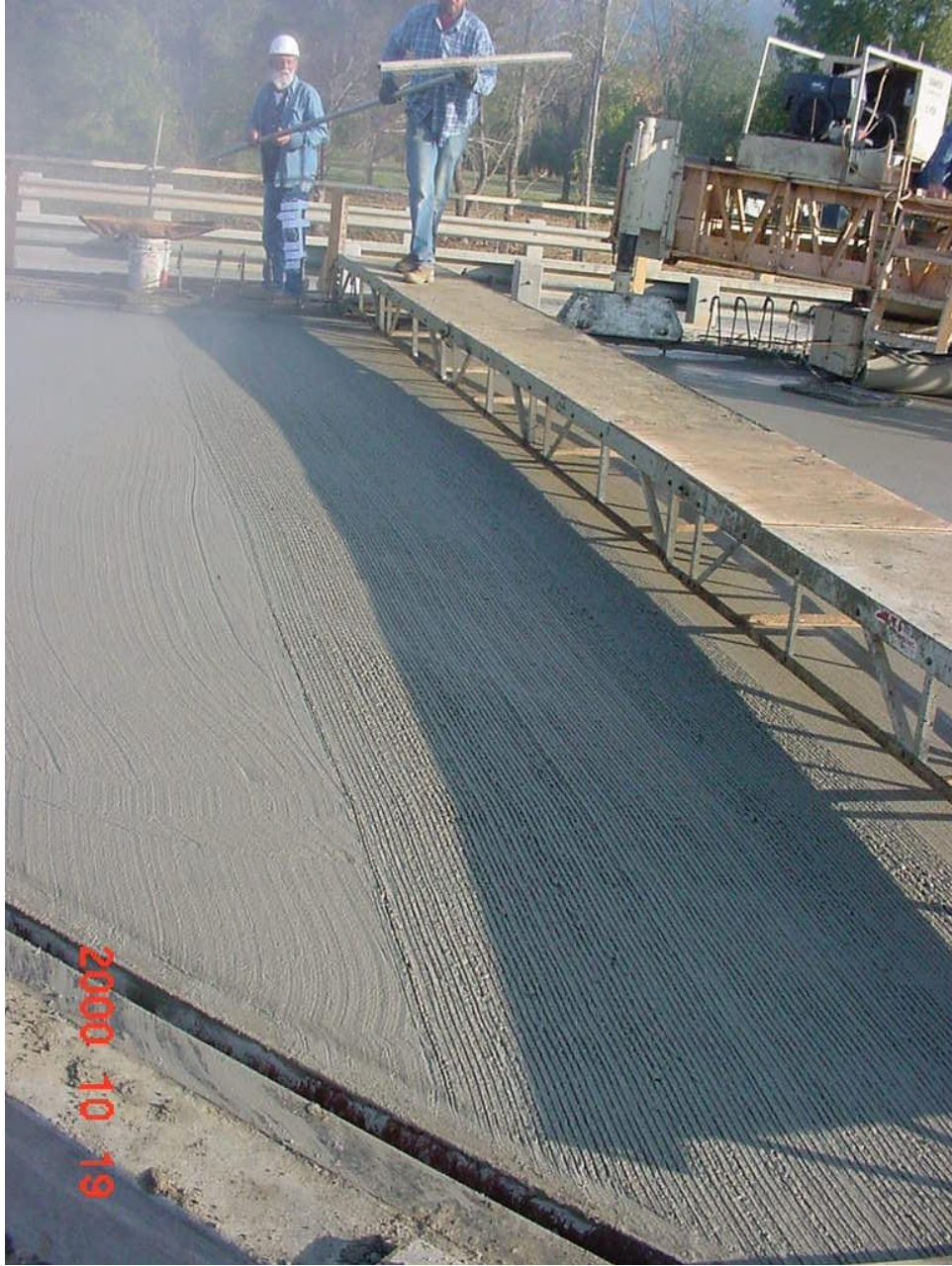
Figure 4a: Tining on Adona Bridge Deck
